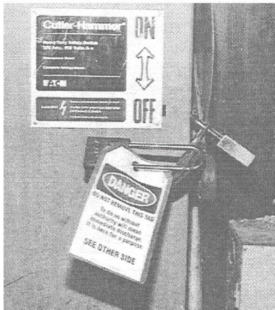
Fig. 3-8. Lock-out tag in place on main disconnect switch located on the machine control panel.
