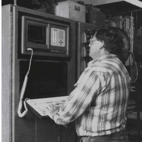
Fig. 5-5. A data acquisition system for monitoring the shot profile can be useful piece of process control equipment.
